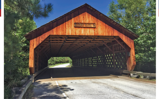
Haralson Mill Covered Bridge, Conyers
